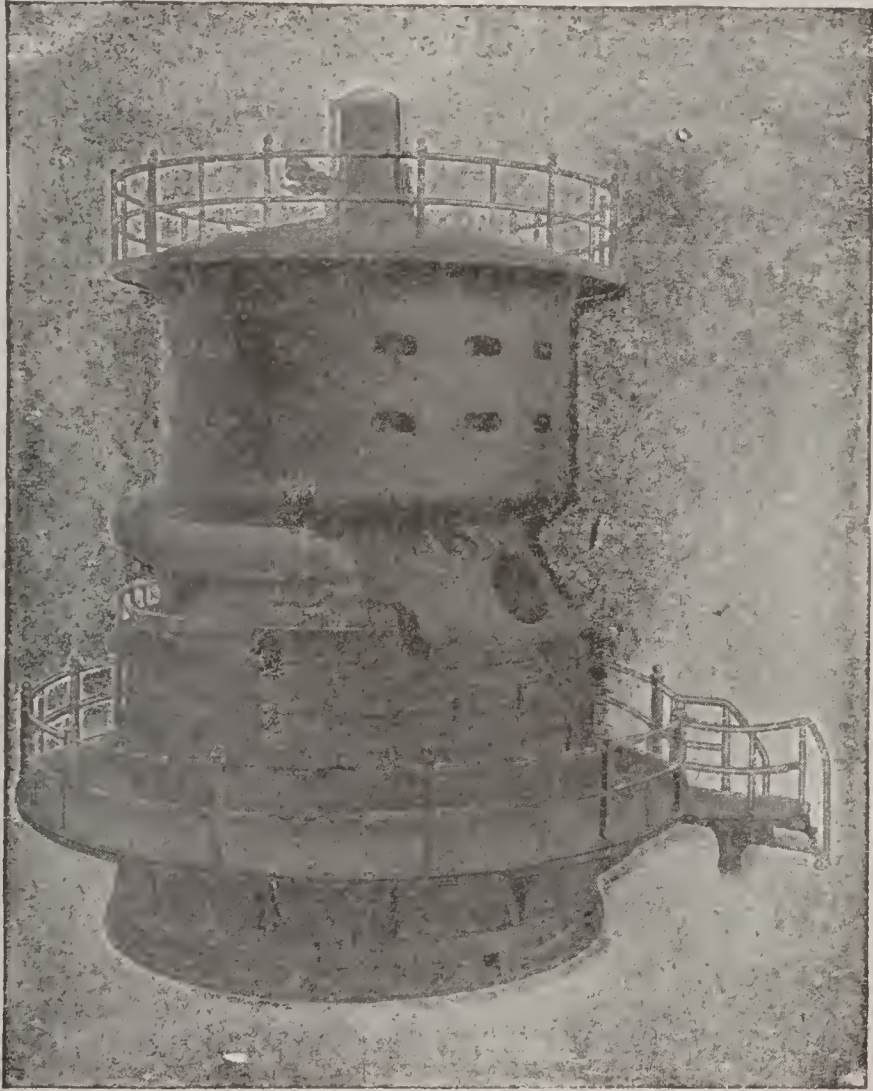
FIG. 193. 5,000 K. W. CURTIS STEAM TURBINE DIRECT CONNECTED TO 5,000 K. W. THREE-PHASE ALTERNATING CURRENT GENERATOR.
